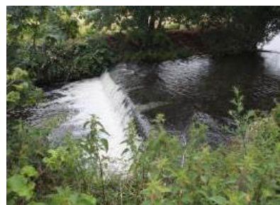
This weir in middle Otter one of a series of four in quick succession acts a partial barrier to fish particularly in low flow condition.
