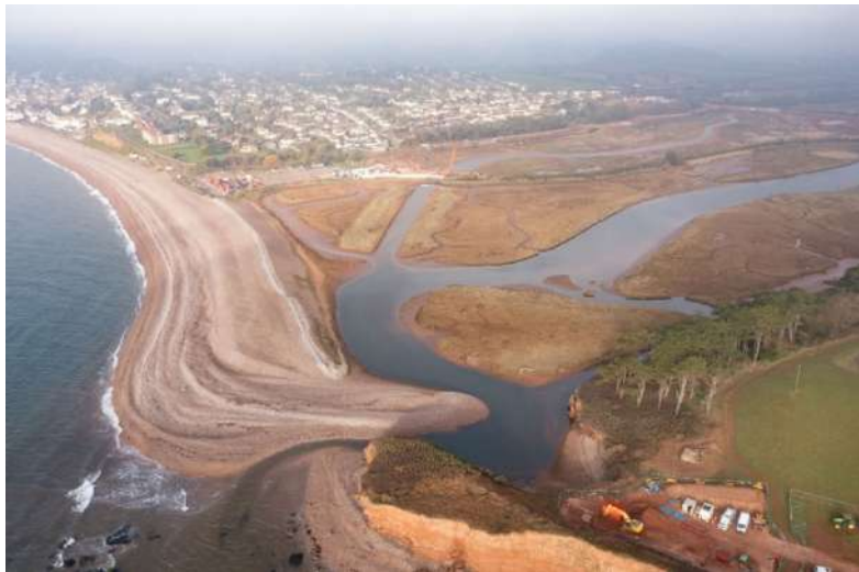
Drone picture of Pipeline Works (photo: SWW)
