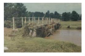
Down river towards Newton Poppleford the footbridge to Harpford survived, but the debris level shows that the river was running at handrail level during the night.
